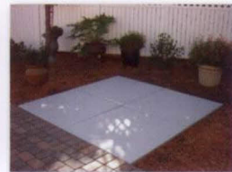
PLACE PADS IN POSITION
