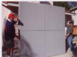
LIFT UP ASSEMBLED PADS
