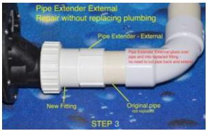
Glue the Pipe Extender External back into the replacement fitting. The overall length of the original pipework remains the same.
