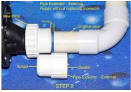
Once the pipe is cut from the faulty fitting, glue the pipe extender OVER the pipe to bring it back to the original length, ready to glue into the replacement fitting.
